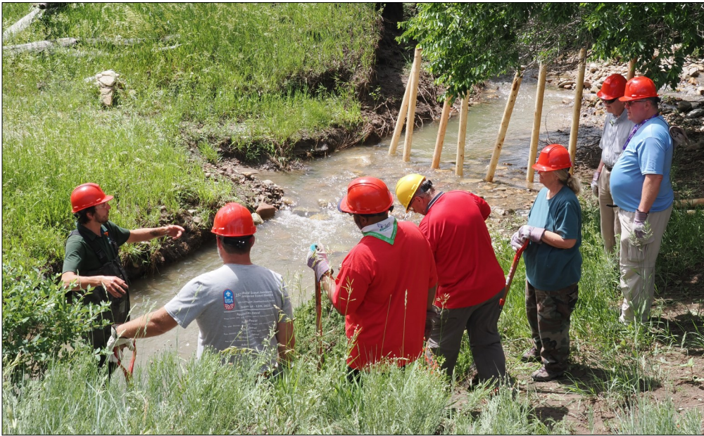
Conservation Department staff explains to a PTC conference class how they will be building an artificial beaver dam behind the stakes driven into Cito Creek. (Tom Baltutis photo.)
