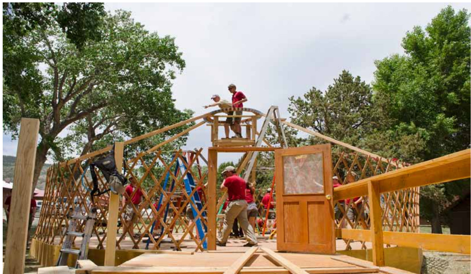
Mark Anderson and Ranger Department Leadership build the framework of a yurt at base camp on Saturday, June 2. The yurt, which will be open in time for the arrival of campers on June 8, will be used as clearance space for the Tooth of Time Traders. MATTEO PROKOSCH/PHILNEWS PHOTOGRAPHER
