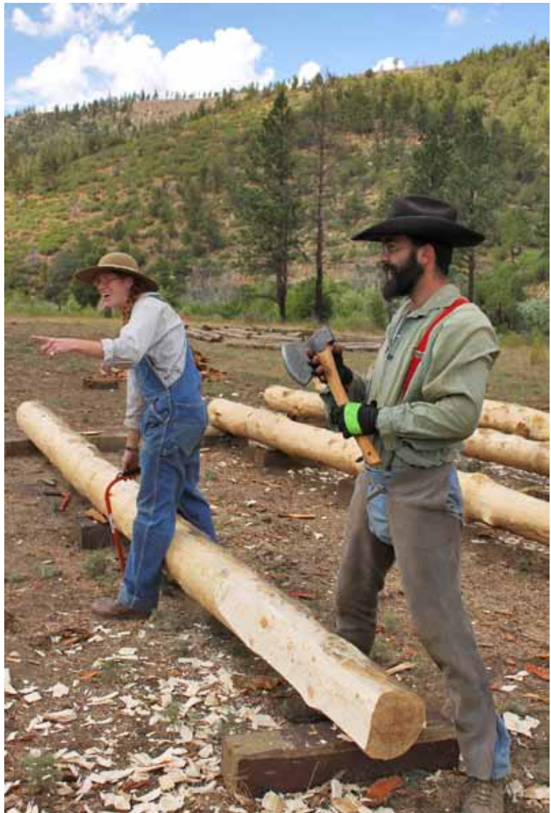
Katharina Stoll and David Bryne hew a log for cabin restoration on Friday, July 6 at Rich Cabins. Stoll and Bryne have been restoring the cabin since the beginning of the summer. CONNOR SPURR/PHILNEWS PHOTOGRAPHER
