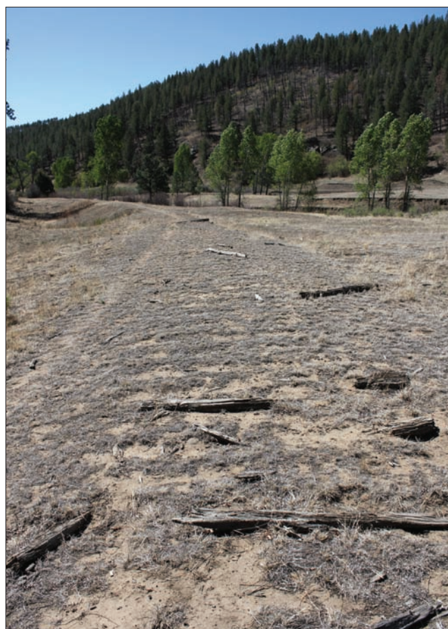
A few of the original wooden ties remain along the original Cimarron and Northwestern Railroad Company Line on Sat., June 1 at Old Camp. One hundred feet of track will be placed along the historic line this summer. CONNOR SPURR/ PHILNEWS PHOTOGRAPHER
