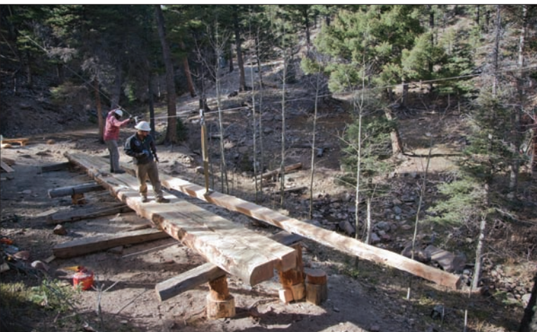
Conservation Department staff move a beam into place on Thurs., Nov. 1 at Cypher's Mine. The bridge, now completed, has been under construction since fall 2012. KATY MOONEY/PHILNEWS PHOTOGRAPHY MANAGER.
