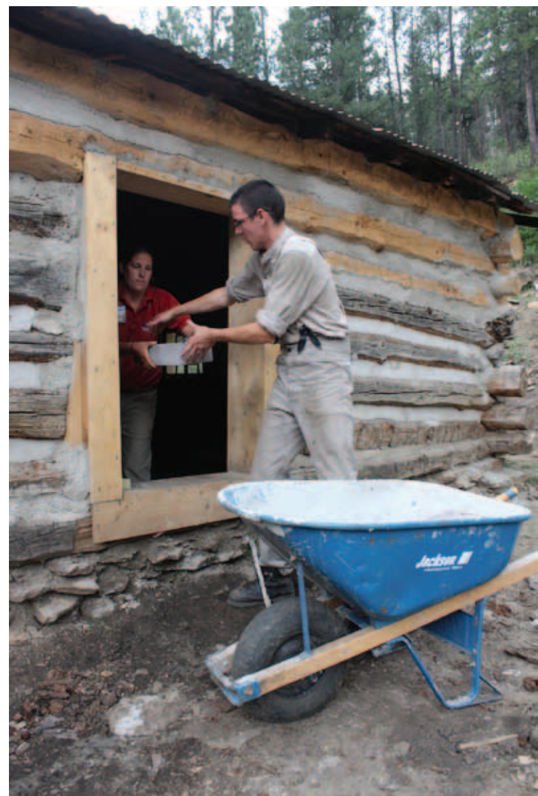
Ranger Dianna Green hands a cinderblock to Cabin Restoration staff Reid Johnston on Tuesday, July 23 at Rich Cabins. The Cabin Restoration staff spend the summer repairing parts of the building so it can be used for program in the future. CONNOR SPURR/PHILNEWS PHOTOGRAPHER
