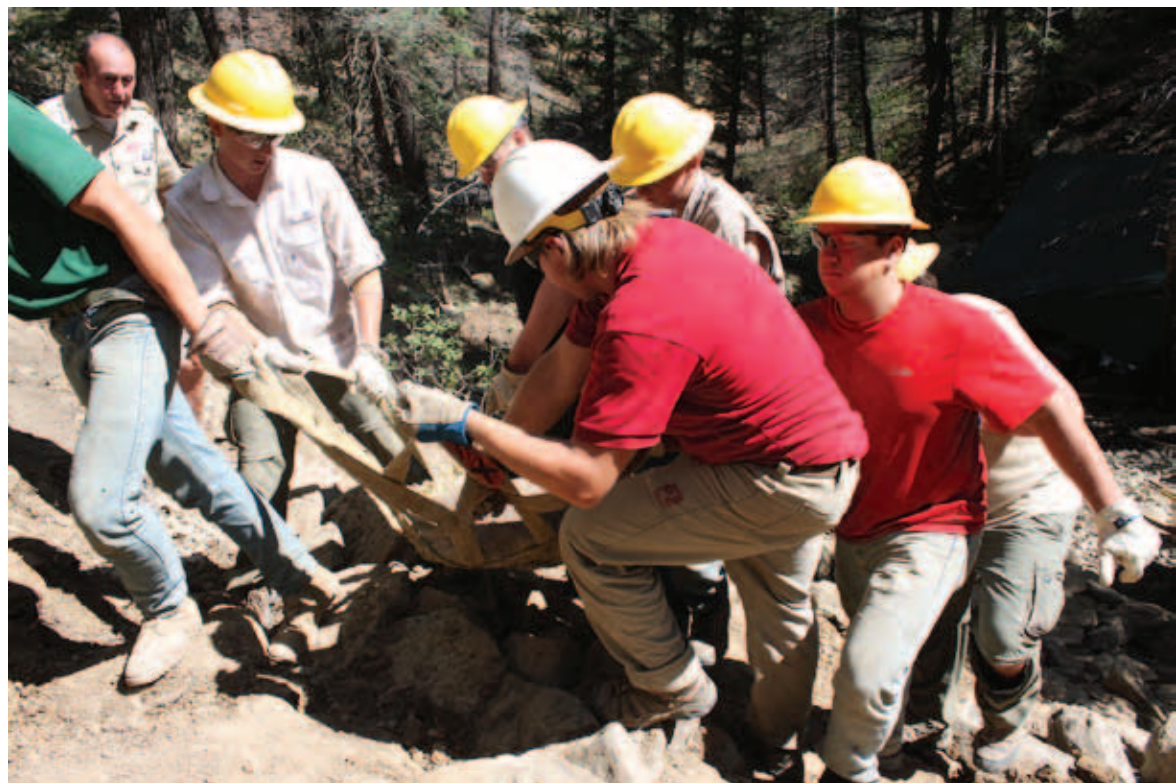
Participants from 713-OA-01 and 2 carry up a boulder to the trail on Thursday, July 18 at Flume Canyon. The OA Trail Crew constructed a rock wall to support a trail that is between ten and twelve feet. CONNOR SPURR/ PHILNEWS PHOTOGRAPHER
