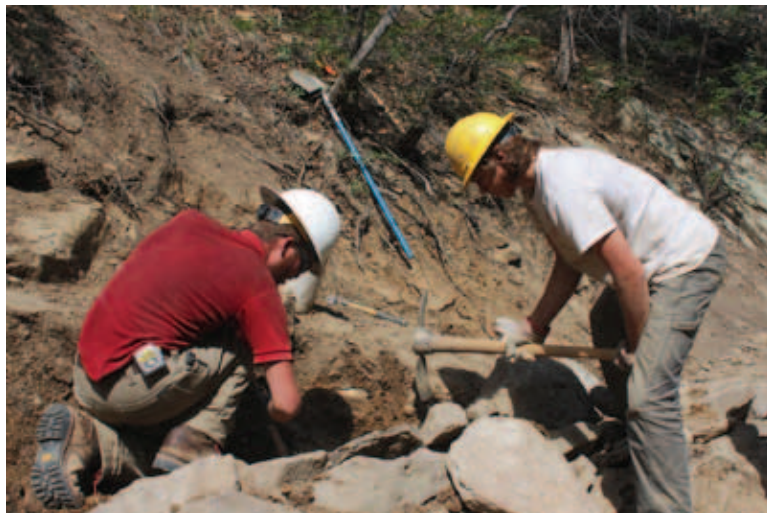
An OA Trail Crew Foreman and Ryan McGunn, a participant from 7130A1, work together to dig out the hillside for the trail on Thursday, July 18 at Flume Canyon. After working on trail, the OA Crews hike on a personal made itinerary through Philmont. CONNOR SPURR/ PHILNEWS PHOTOGRAPHER
