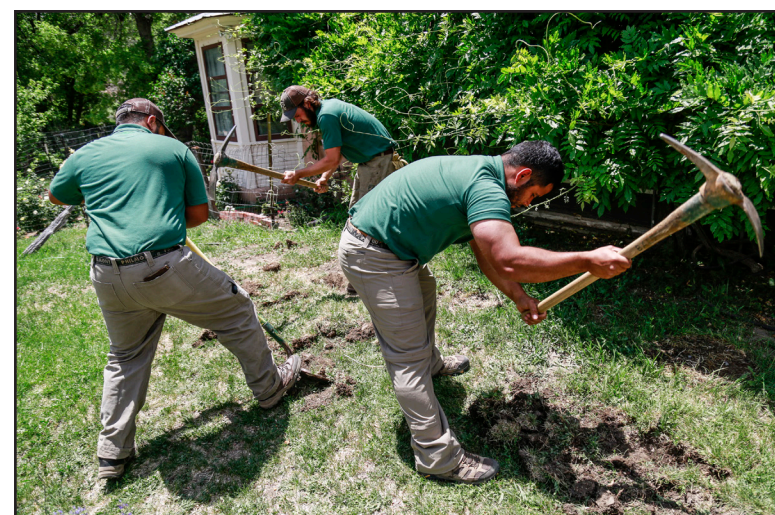
Members of Cabin Restoration work to uncover the original stone patio at Chase Ranch. Jess McClelland/MPS Photographer
